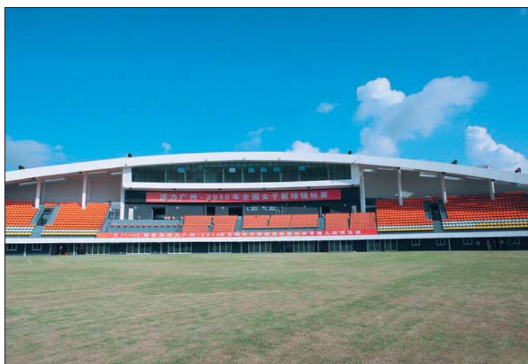
Guangdong International Cricket Stadium © Travis Pittman
